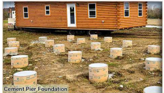
Cement Pier Foundation
