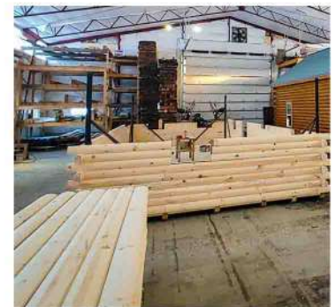
Cabin under construction
